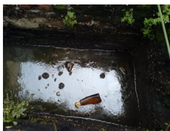
Wastewater in Namdinh Silk Co.
