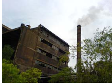
Old factory without improvement
