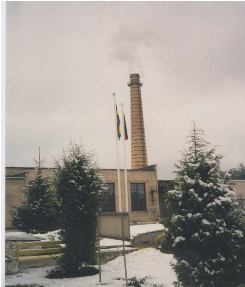
Fig. 7.1. Ignalina Biofuel Boiler Plant
