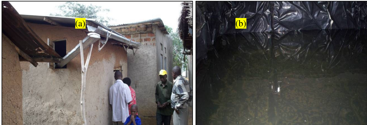
Figure 7: (a) the outside view of the water store and (b) inside view of the water store
