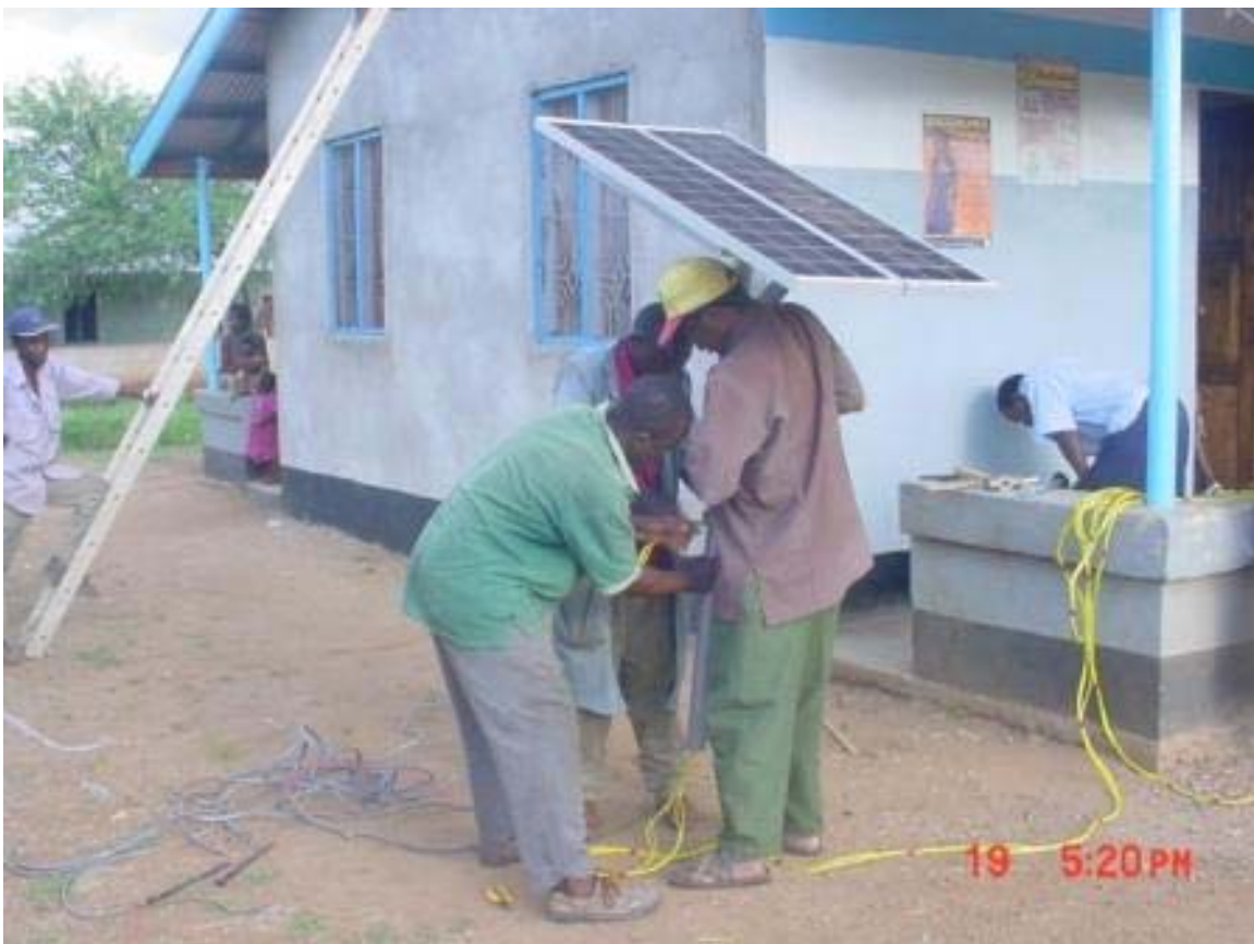
Plate 2: Rural technicians installing a solar PV system at Ngasamo dispensary, Magu.
